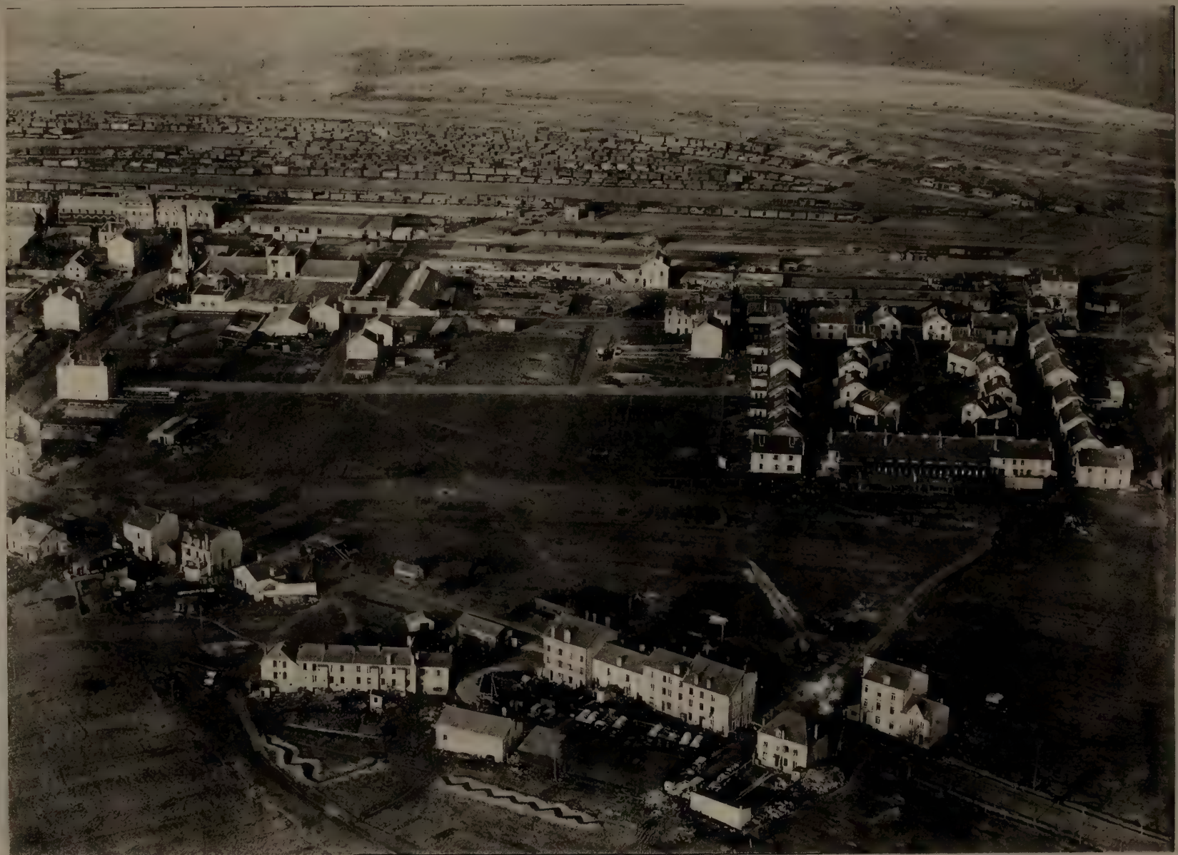
Aerial Picture of Railhead at "Conflans," Notice how plain the Trenches and Trucks in the Foreground show up by not being Camouflaged.
